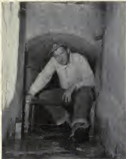
JACKING UP THE GATE of the Pleasant Valley Dam meant that Reynold L. Johnston, manager of the Pleasant Valley Irrigation Co., had to crawl the length of the 240-foot tunnel with heavy equipment to renovate the outlet gate. Photo by Stanley Rosmussen, Region 1 photographer. Artist's impression of Reynold at work by Lloyd Chellman, Graphics Section, Washington, D. C.
